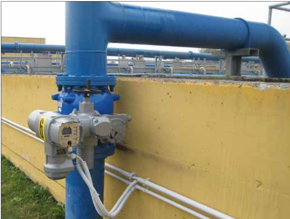
Fig.1 - Plunger valve for controlling air flow inside oxidation tanks.
