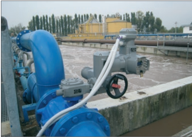
Fig.1, 2 - Plunger valve for regulating air flow into a nitrification tank: the valve is equipped with an electrical actuator.
