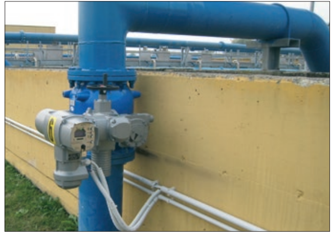
Fig.1, 2 - Plunger valve for regulating air flow into a nitrification tank: the valve is equipped with an electrical actuator.
